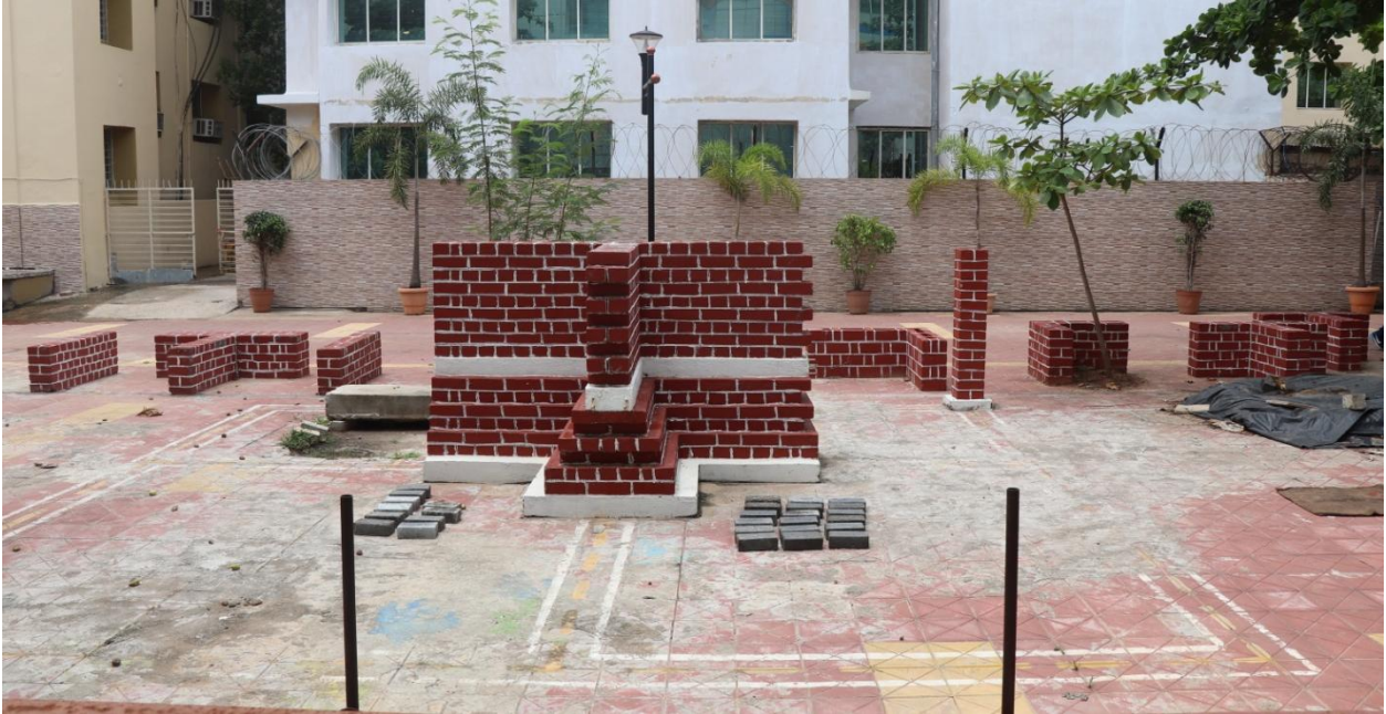
Overview image of the Masonry Demonstration Laboratory
