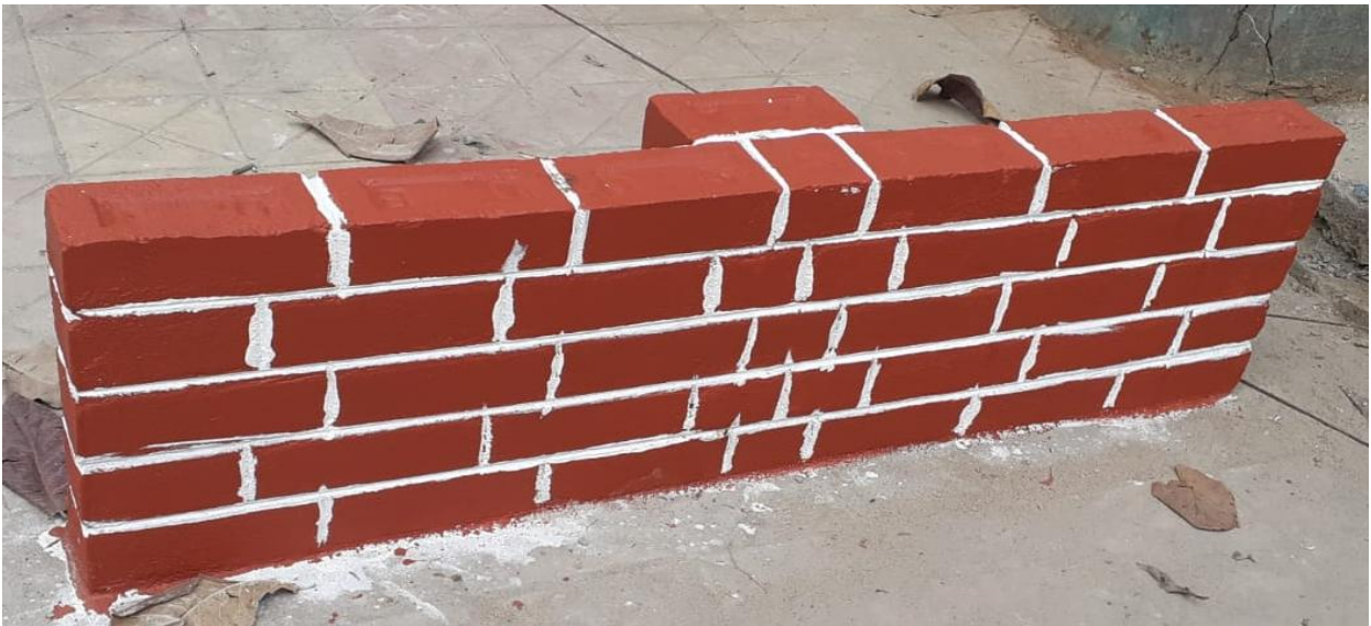
HALF BRICK THICK STRETCHER BOND
